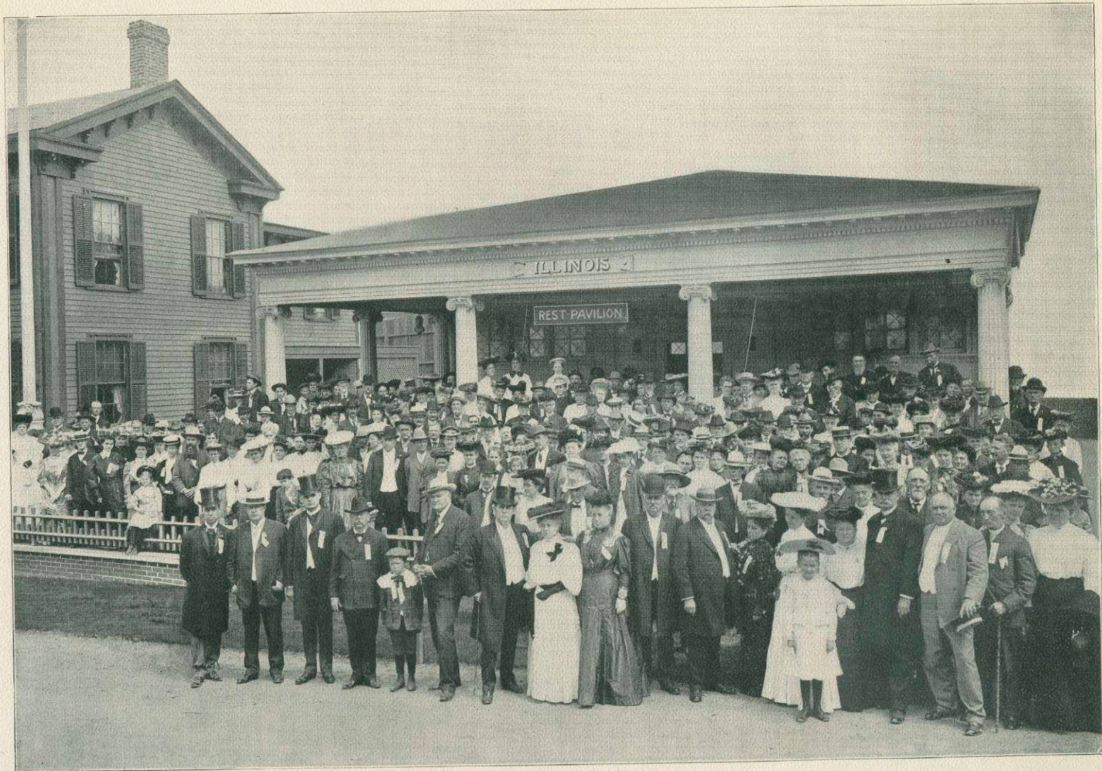
Group of Illinoisans on Rest Pavilion, Illinois Day
