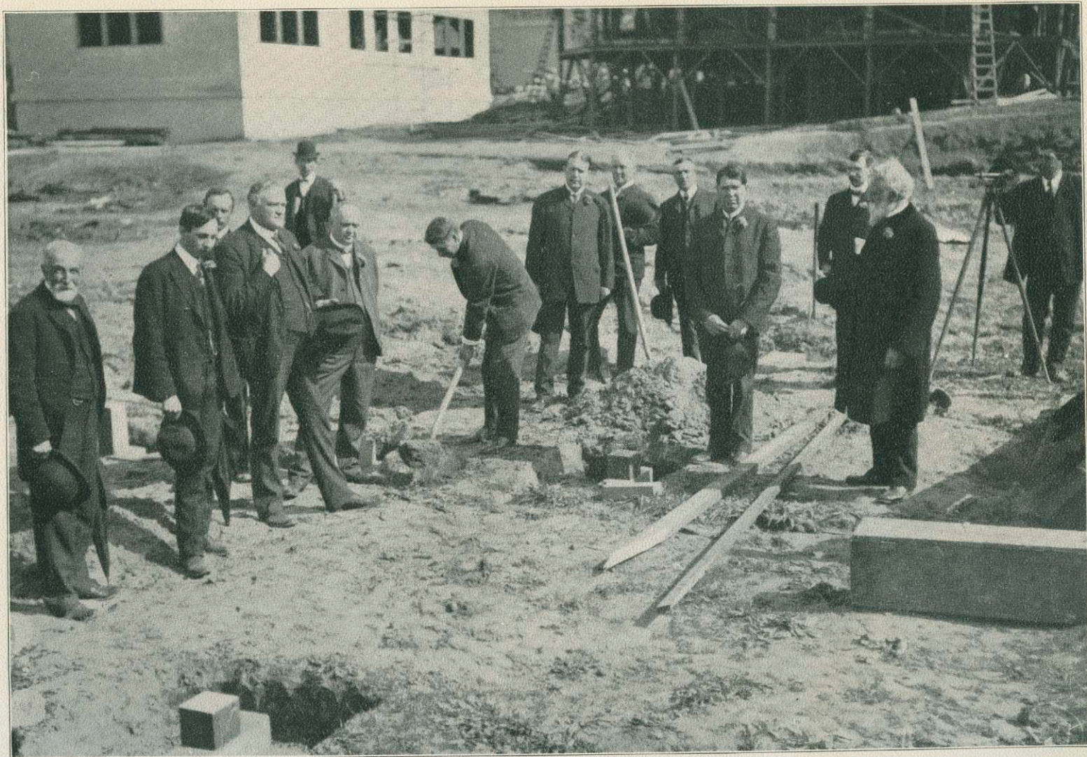
Breaking Ground for the Illinois Buildings, May 6, 1905
