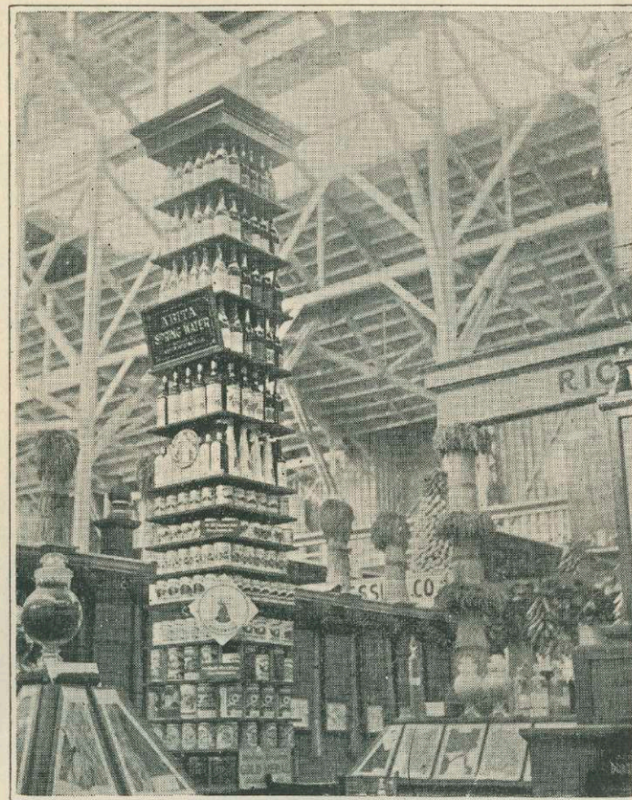
Interior view of tower of mineral water, etc.
