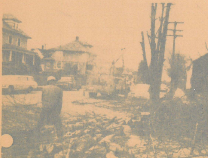
DEBRIS CLEANUP 3530 North Kerby
