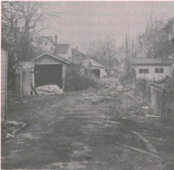
PAVING OF ALLEYS
