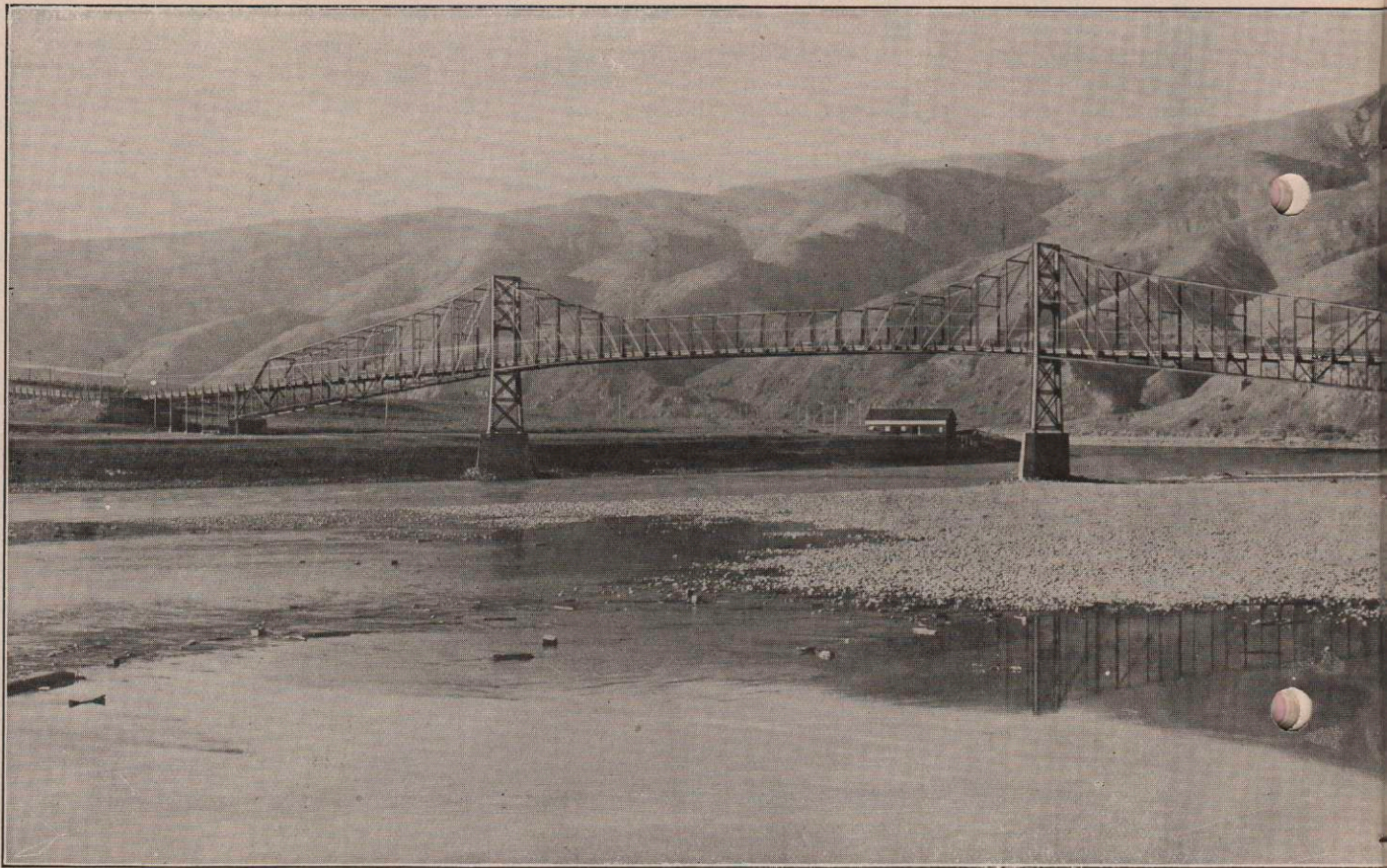
STEEL BRIDGE CONNECTING LEWISTON-CLARKSTON
