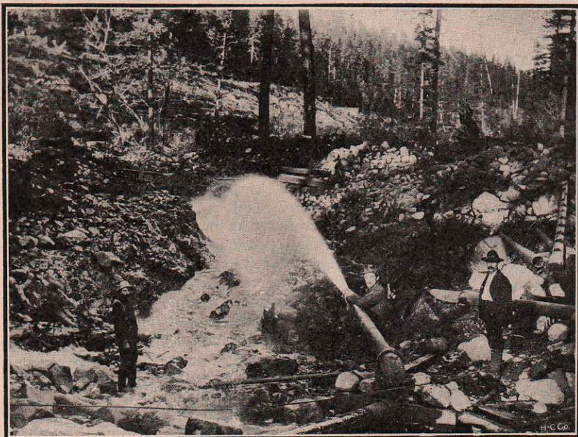
Hydraulic Mining—Pipeman and a "giant" stream.
